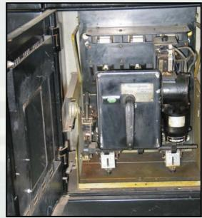
Circuit Breaker used as Motor Starter
