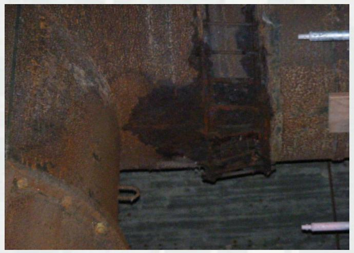
PS#2 discharge pipe coupling ruptured. Discharge pipe supported by scaffolding
