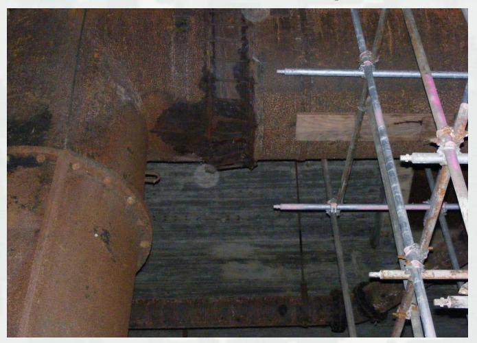
PS#2 discharge pipe coupling failing! Pipe supported by scaffolding
