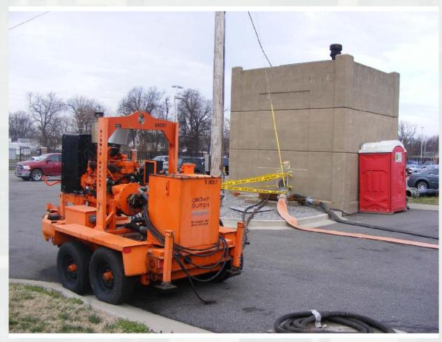
PS#9, Pump Temporary Pumps added to the station to offset lost pumping capacity at this station.
