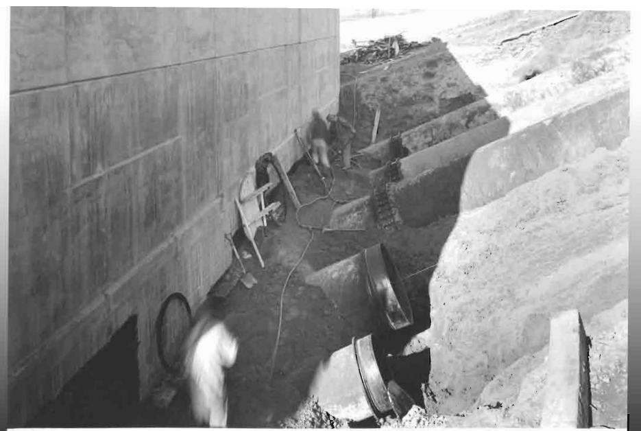
WAR DEPAPTMENT U. S. ENGINEER OFFICE LOUISVILLE DISTRICT Paducah Flood Protection Project (Pumping Plants) - Ohio Piver. For protection of Paducah, Kentucky. View on downstream riverside of Plant No. 2 showing installation of discharge pipes. Contract No. W559eng-5785, 27 Jan. 1942. Midland Constructors, Inc., contractor.
