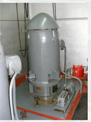
PS#9, Pump No. 2 has a broken drive shaft that causes this pump station's output to be reduced by 50%.
