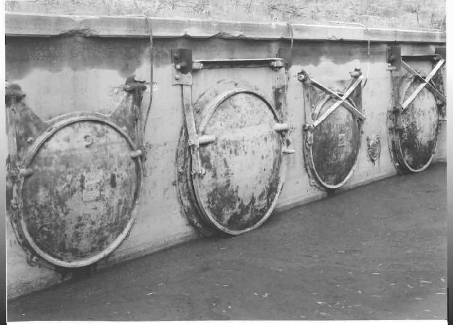
LOUISVILLE DISTRICT, CORPS OF ENGINEERS, U. S. ARMY. Date: 8 June 1950. File No. 24517 Flood Control--Paducah, Kentucky, Ohio River, Paducah Flood Protection Project, Pumping Plant No. 2. View showing damaged 48 inch and 60 inch flapgates on pump discharge pipes.
