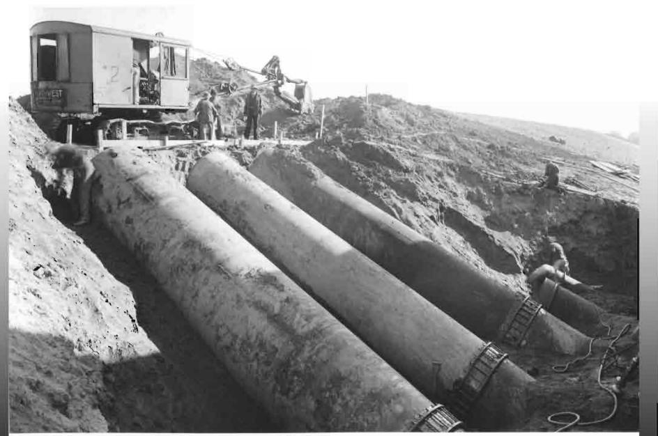
WAR DEPARTMENT U. S. ENGINEER OFFICE LOUISVILLE DISTRICT Paducah Flood Protection Project (Pumping Plants) - Ohio River. For protection of Paducah, Kentucky. Partially completed installation of discharge pipes on landside slope of levee at Plant No. 2. Contract No. W559eng-5785, 27 Jan. 1942. Midland Constructors, Inc., contractor.
