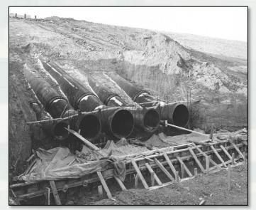
Photo Circa 1949; PS#2 Discharge pipes – 60" dia, 48" dia, 30" dia
