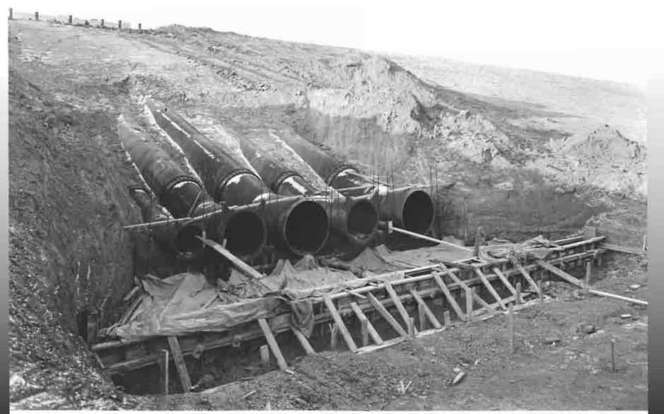
WAR DEPARTMENTU. S. ENGINFER OFFICELOUISVILLE DISTRICTPaducah Flood Protection Project (Pumping Plants) - Ohio River. For protection of Paducah, Kentucky.<br/>Discharge pipes at Pumping Plant No. 2, before backfilling and placing of headwalls. Contract No.<br/>W559eng-5785, 27 Jan. 1942. Midland Constructors, Inc., contractor.Contract No.
