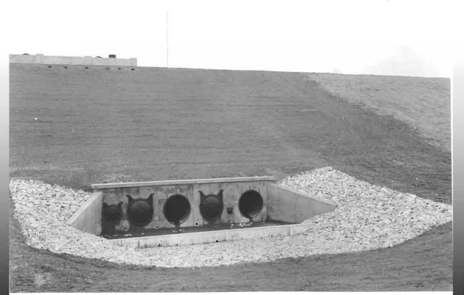
WAR DEPARTMENTU. S. FNGINEER OFFICELOUISVILLE DISTPICTPaducah Flood Protection Project (Pumping Plants) - Ohio River. For protection of Paducah, Kentucky.<br/>Discharge Headwall and Riprap at Pump Plant No. 2, complete except for installation of two gates.<br/>Contract No. W559eng-5785, 27 January 1942. Midland Constructors, Inc., contractor.
