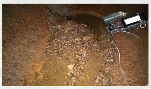
Photo November 2015, PS#2 Discharge Pipe Severely eroded pipes with voids
